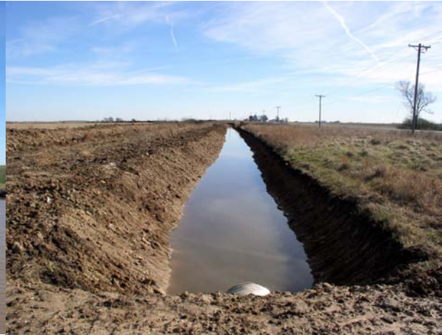
Surface Drain, Main or Lateral
