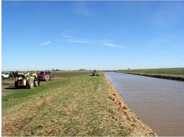
Irrigation Reservoir – Excavated
